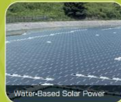
Water-Based Solar Power
